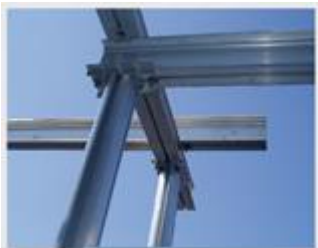
Supershore Typical Connection
