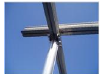
Supershore Typical Connection
